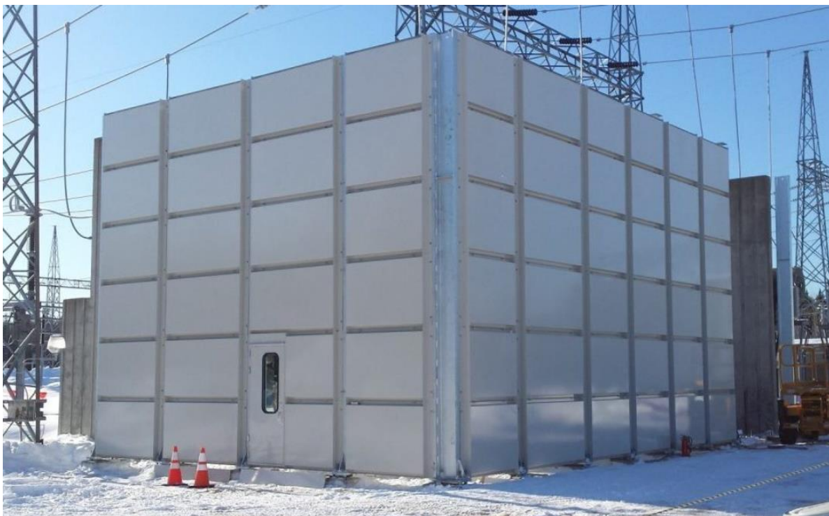
Plate 4.4 A typical steel panel noise enclosure surrounding a transformer.
