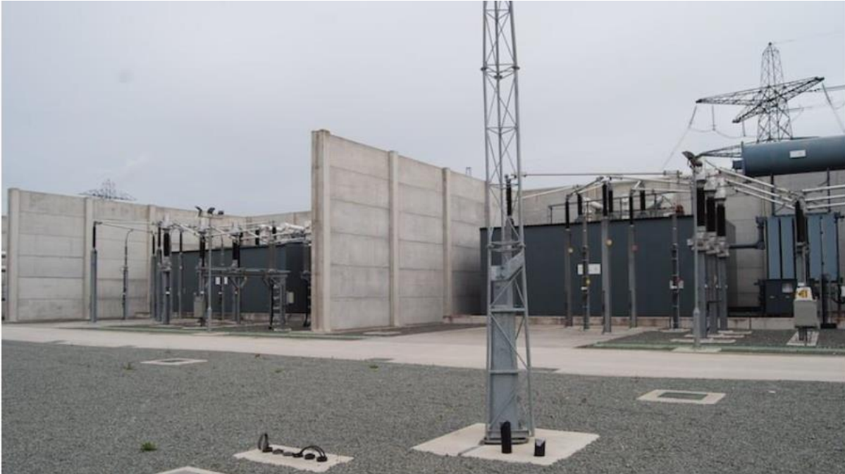
Plate 4.3 A typical transformers in acoustic enclosures (grey metal boxes) with concrete fire walls
