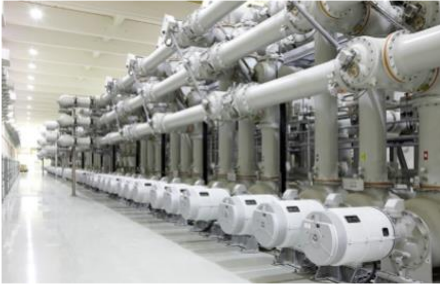
Plate 3.2 Typical 400kV GIS switchgear
