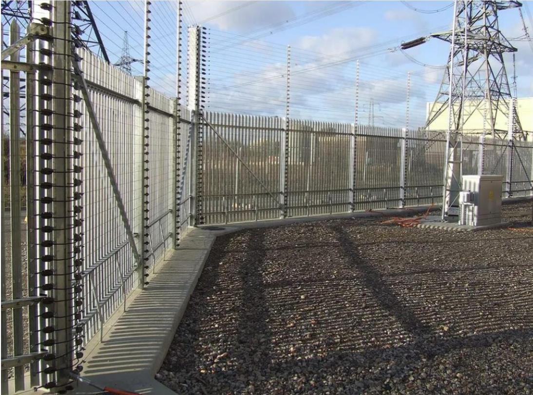
Plate 4.5 Typical examples of high security external fencing
